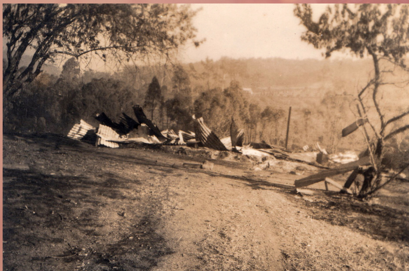
Burnt Aldersyde Road Hutchison house (now number 53 Aldersyde Road) 8 February 1940. House was built about 1914 for Arthur and his bride Stella.
